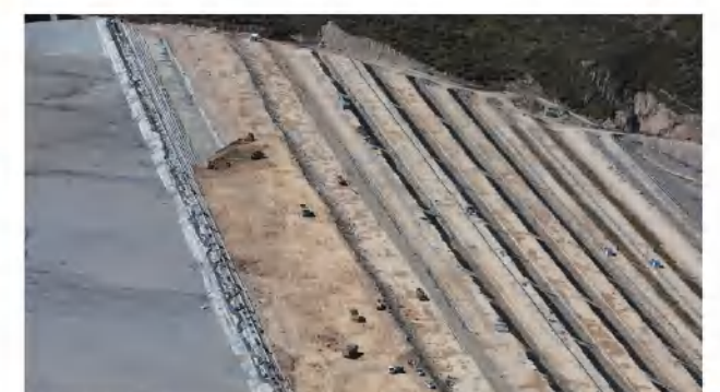
模袋法尾矿堆坝技术 - 西藏华泰龙矿业果郎沟尾矿库 Technology of tailings damming with geofabriform method - guolanggou tailings pond of huatailong mining in Tibet
