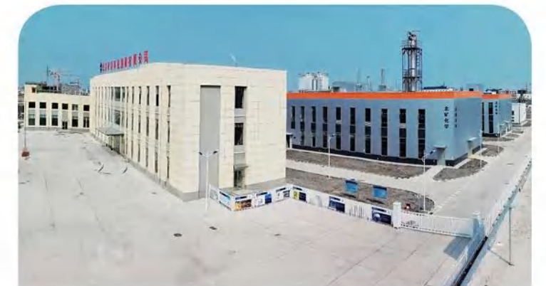
立式砂仓高浓度膏体充填料浆制备系统 Vertical sand silo high-concentration paste backfill slurry preparation system
