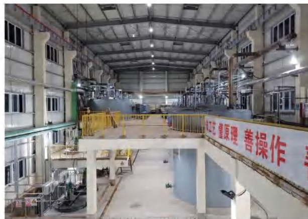
紫金铜业铜冶炼资源综合利用及无害化处置工程 Comprehensive utilization and harmless disposal project of copper smelting resources in Zijin Copper
