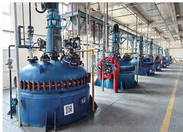
北矿化学沧州工厂生产线及调度中心 Production line and control center of BGRIMM Chemical Cangzhou Factory
