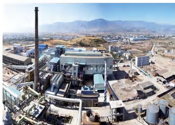
康西铜业 5 万吨铜侧吹熔池熔炼项目 50,000t/a double side-blown bath smelting project in Kangxi Copper Corporation, China
