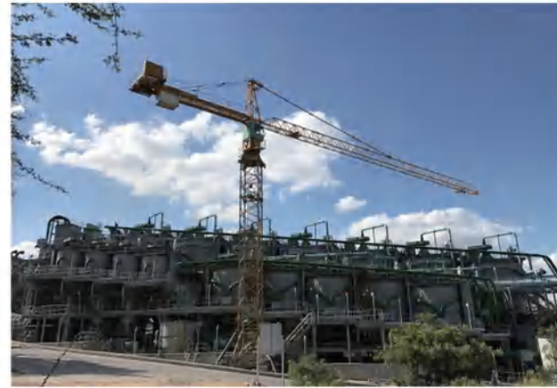
南非帕拉博拉铜矿浮选厂 EPC 工程 EPC project of flotation plant of Phalabora copper mine in South Africa
