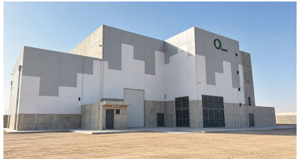
Damac Lagoons DEWA Substation
