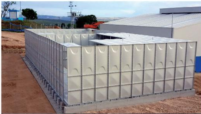
■ Completion of Side Panels
