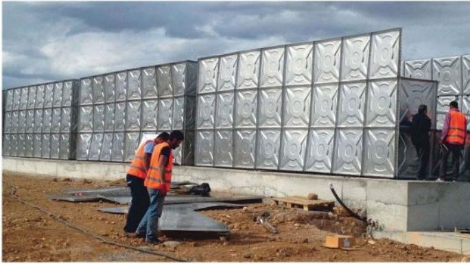
■ S.Urfa / Harran Refugee Camp - AISI Steel Water Tank 2400 M 3
