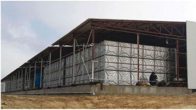
■ K.Maras / Sivrice Container Town - AISI Steel Water Tank 2400 M 3
