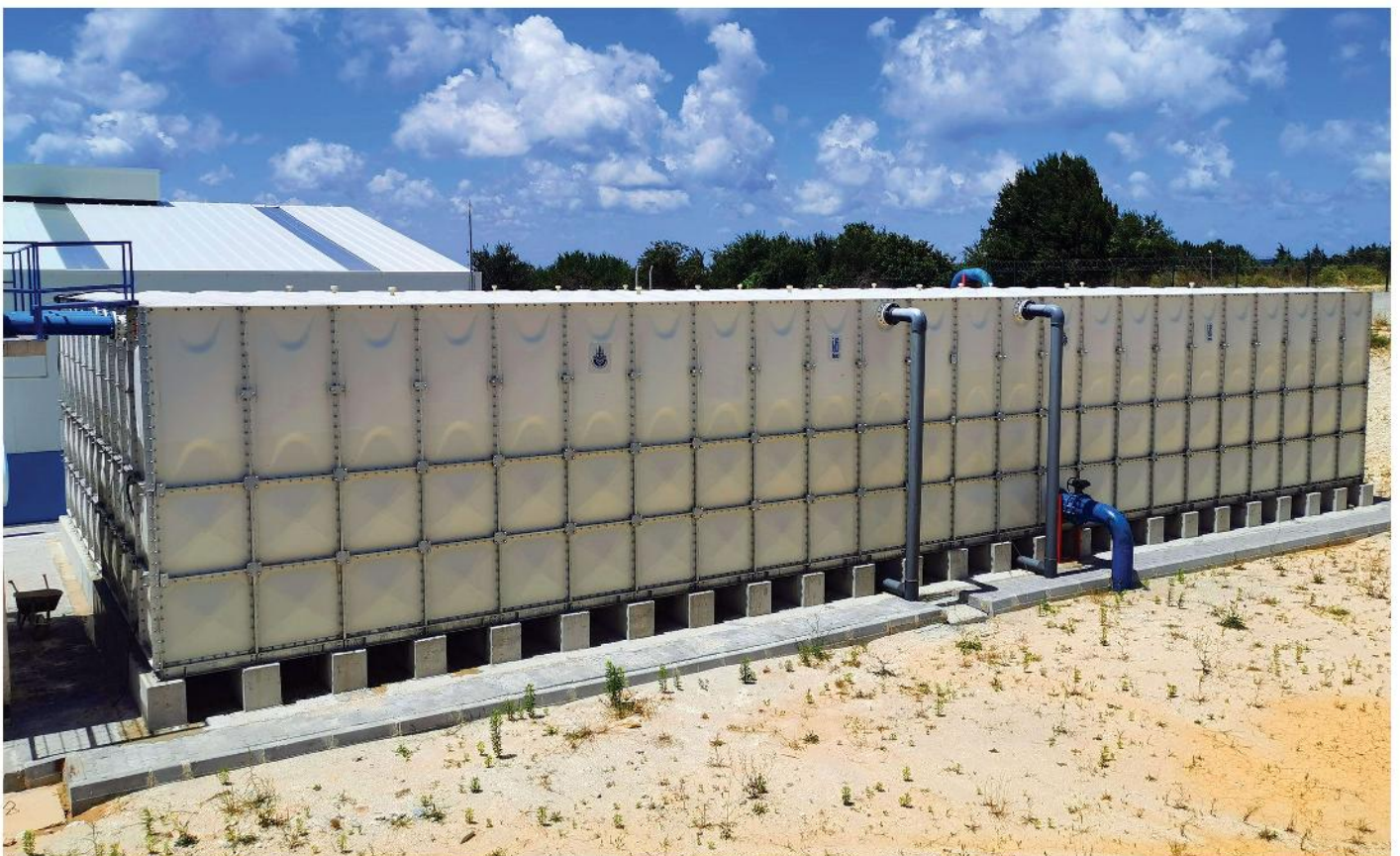
■ Commissioning of the Water Tank
