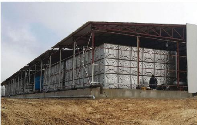
K.Maras / Sivrice Container Town - AISI Steel Water Tank 2400 M 3
