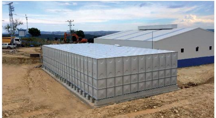
■ Completion of Top Roof Panels
