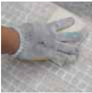
Clean the tile surface
