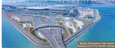
Beijing-Zhangjiakou High-Speed Railway Line for the Winter Olympics
