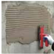
Apply 3TREES Tile Adhesive on the wall
