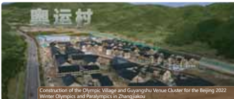
Construction of the Olympic Village and Guyangshu Venue Cluster for the Beijing 2022 Winter Olympics and Paralympics in Zhangjiakou
