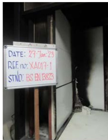
After Fire Test
