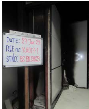
After Fire Test
