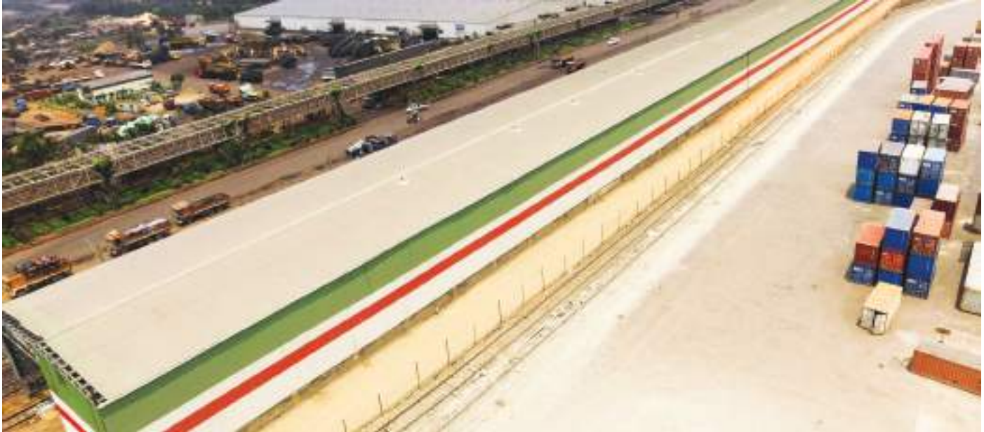
1 KM long Automatic Conveyor PEB | KPCL | Krishnapatnam, AP | Area: 2,51,000 SFT
