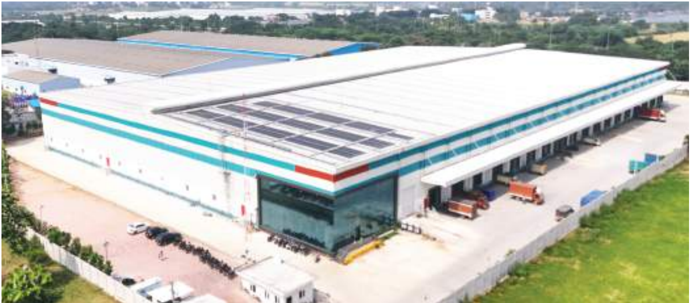
Ware House for Tata Croma | Medchal, Telangana | Area: 1,80,000 SFT (Developer – S. Naveen Chandra Reddy)
