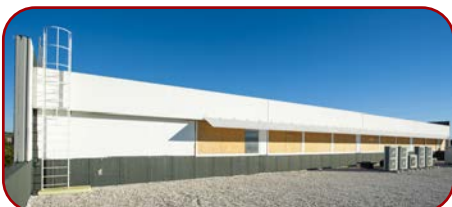
Roof Top Plant Rooms
