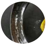
Outer Race Failure
