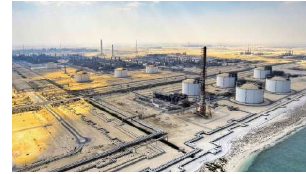
NFE ONSHORE PROJECT - ONGOING
