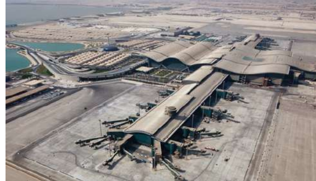
HAMAD INTERNATIONAL AIRPORT - COMPLETED
