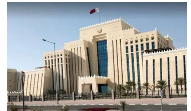
MINISTRY OF INTERIOR - HQ - COMPLETED
