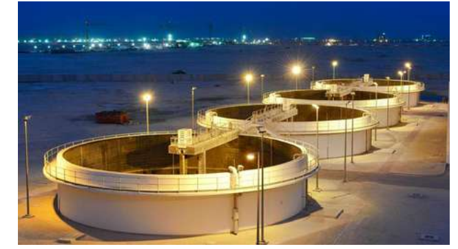
LUSAIL WATER TREATMENT PLANT - COMPLETED
