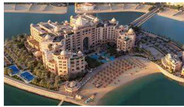
MARSA MALAZ HOTEL THE PEARL - COMPLETED
