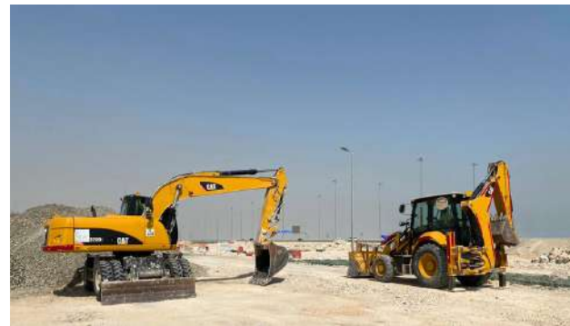
ROADS AND INFRASTRUCTURE WEST OF AL MESHAF - ONGOING
