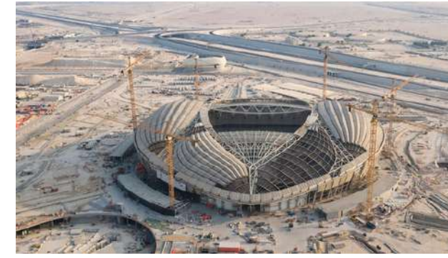
AL WAKRA STADIUM - COMPLETED
