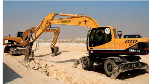
TSE LINE CONNECTION TO ASHGHAL TSE - ONGOING
