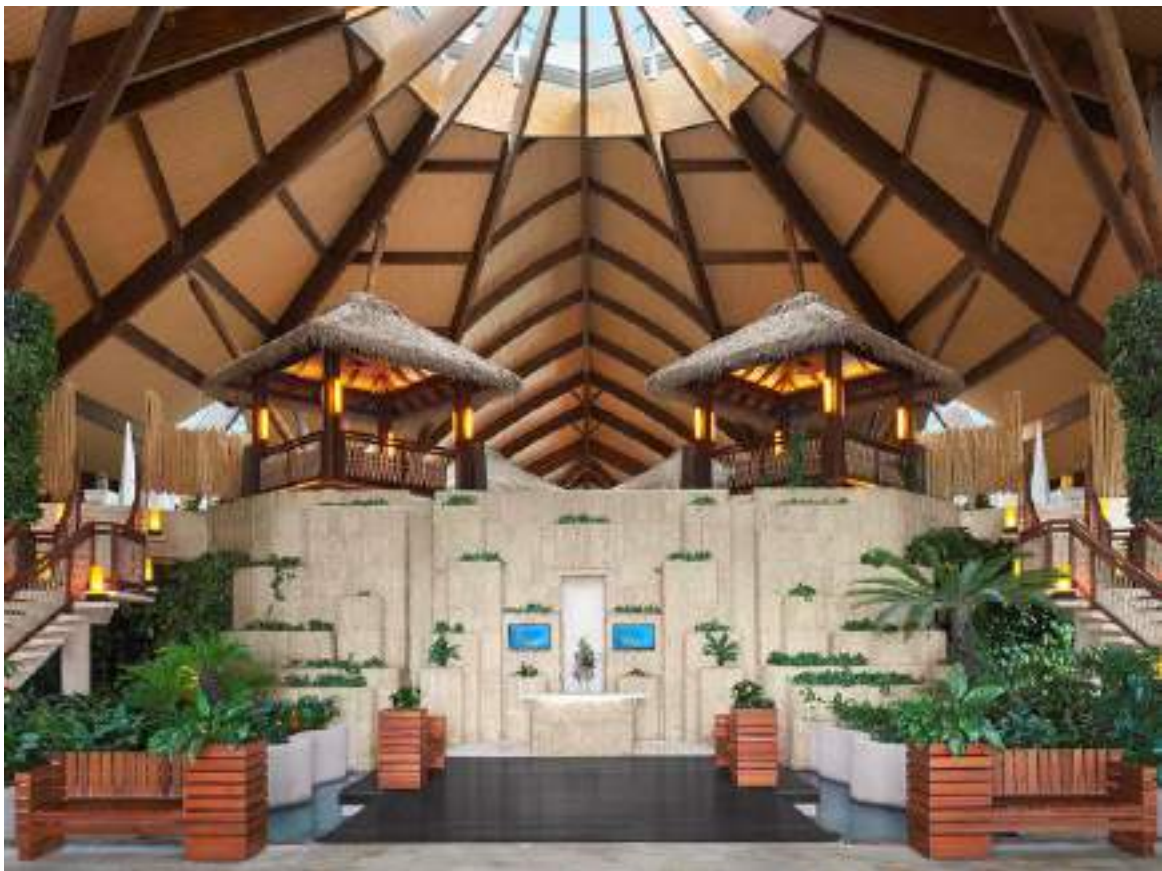
Doha - Banana Island (Qatar) Wellness center Glulam beams with Résix® connections 48 m long Sapisol sandwich panel
