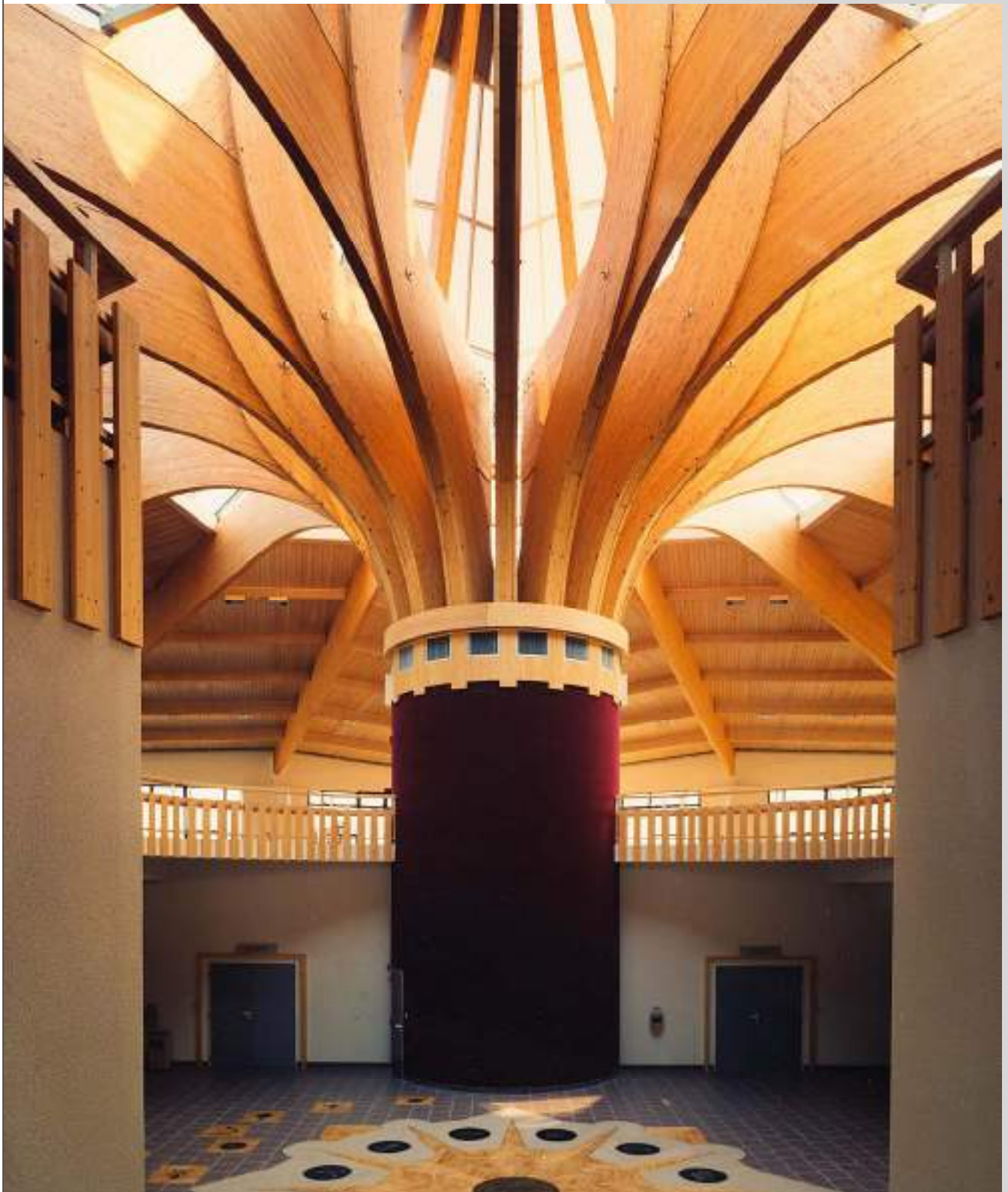
Micropolis Besançon (France) Convention Center 80m in diameter, 2m high beams
