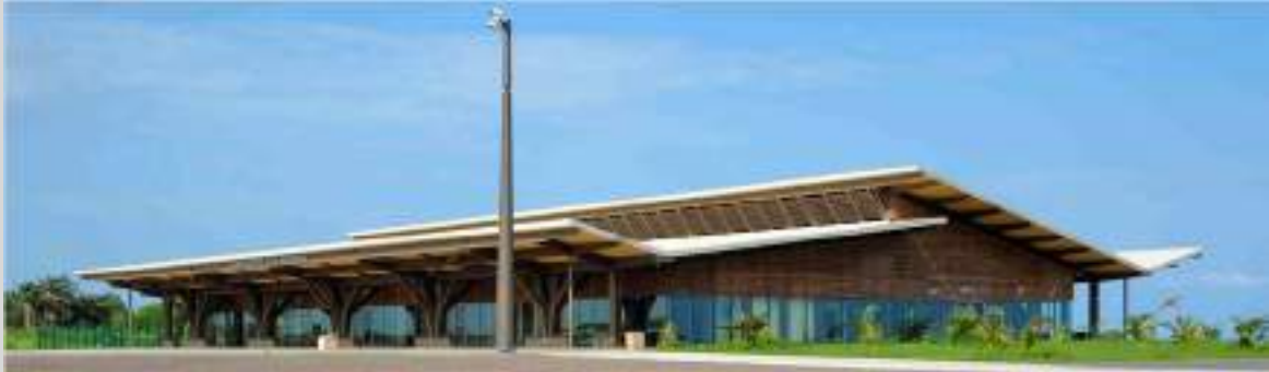
Annobon island (Equatorial Guinea) Airport Terminal Glulam structure with Résix® connections Sapisol® roofing with special acoustic profile
