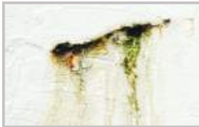
Leakage through cracks on exterior walls
