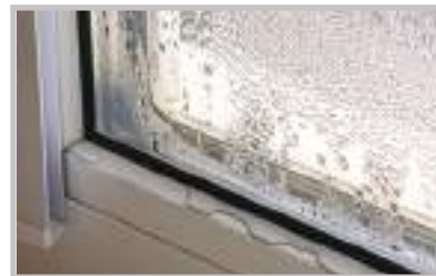
Leakage through window gaps
