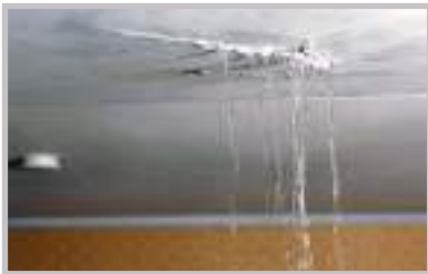
Leakage through roofs
