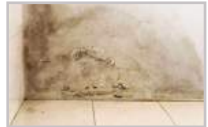
Leakage problems in bathroom
