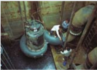
Azizia Pumping Station Place: Saudi Arabia (Dammam) Products: KSE 650 pumps ( 3 x 650 KW ) Application: Waste Water Maangement
