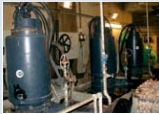
RAKA Pumping Station Place: Saudi Arabia Products: Submersibles pumps ( 2 x 230 KW) Application: Sewage Treatment Plant
