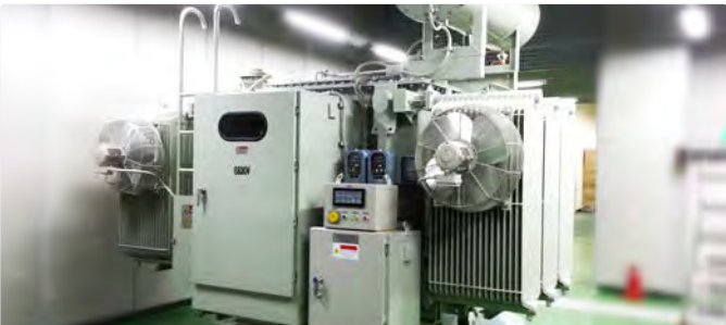
e. Distribution TR 6MVA-6600V-575V
