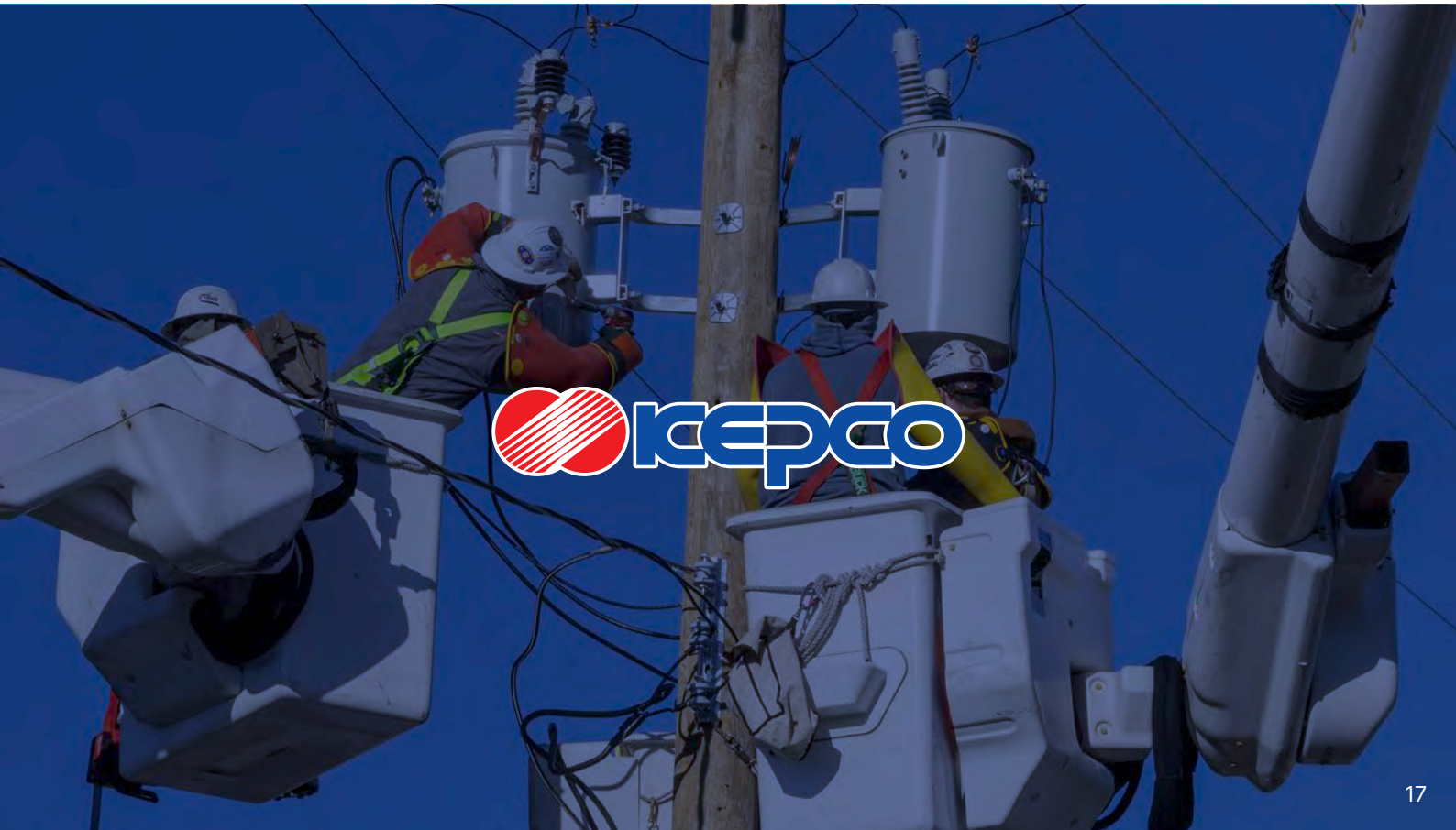
c. High Efficiency Pole TR 10-167kVA
