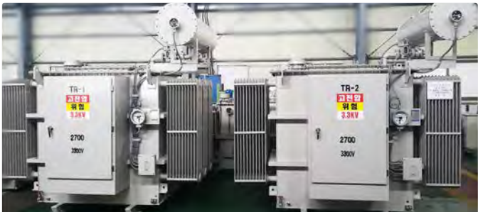
f. Distribution TR-2700kVA-3300V-460V
