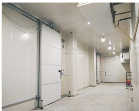
Cold Storage Doors
