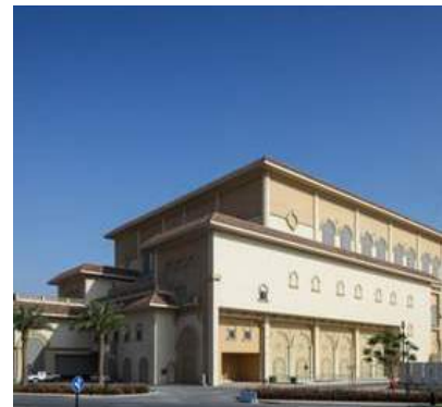
Sea Water Desalination Plant for Pearl, Qatar MEED's Quality Awards Projects for 2012
