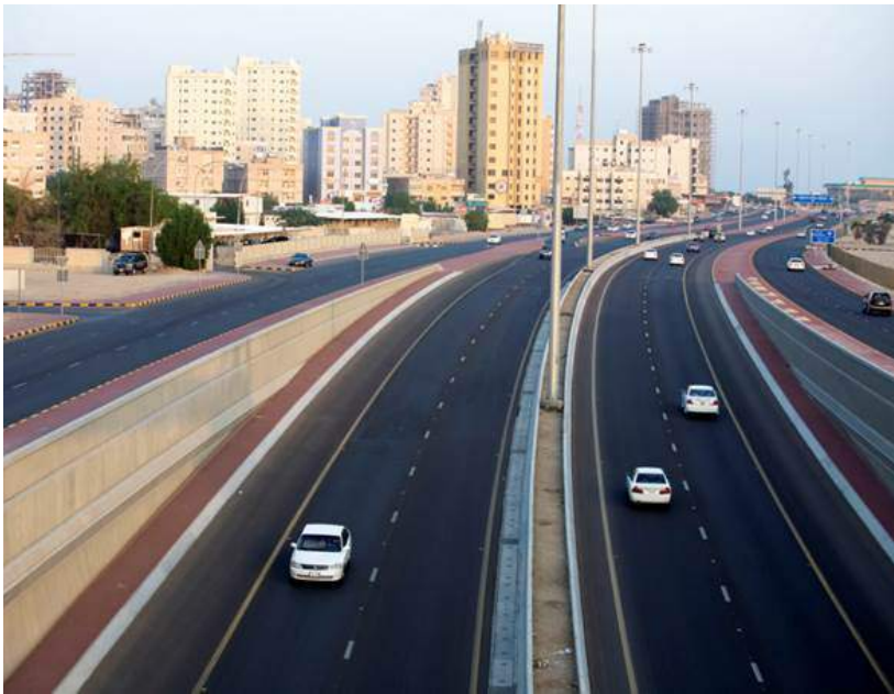
5 th Ring Road, Kuwait Outstanding Design Award, 2010 recognition by Ministry of Public Works
